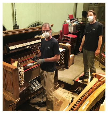
Skilled technicians removed the console from the organ, lowered it on a lift from the choir loft to ground level and transported it to the Casavant workshop in St-Hyacinthe.
