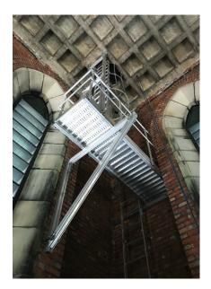
The catwalk between the interior ceiling and exterior roof has been fortified and a special ladder installed to provide safe access to the bell tower.
